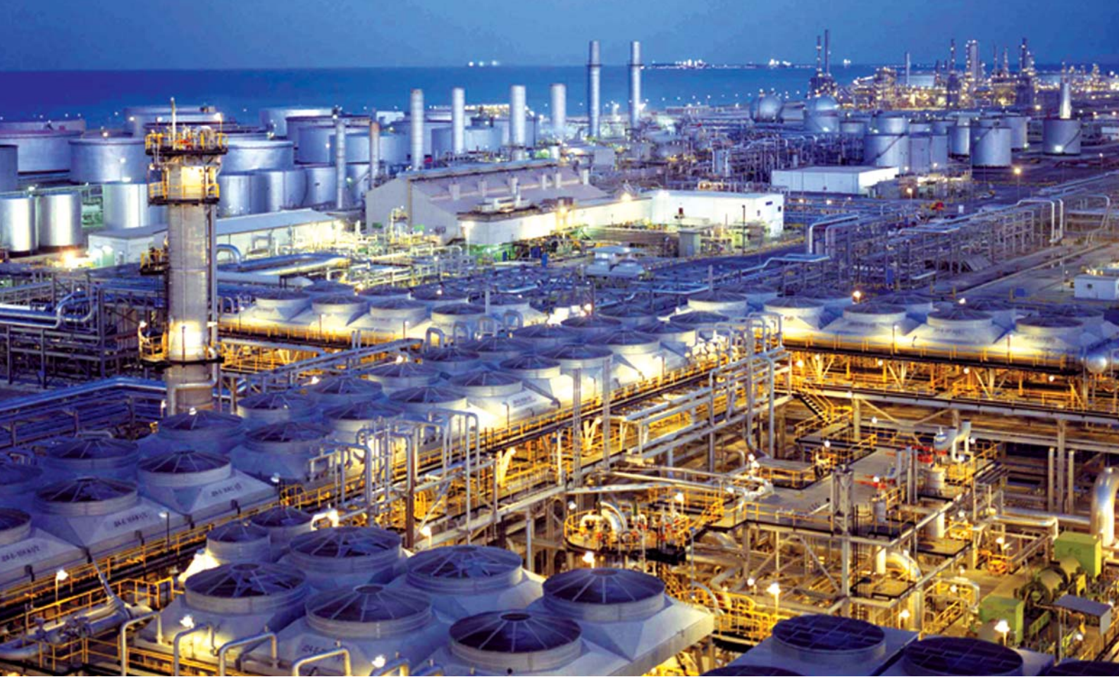
Oil and gas plant in the Gulf
